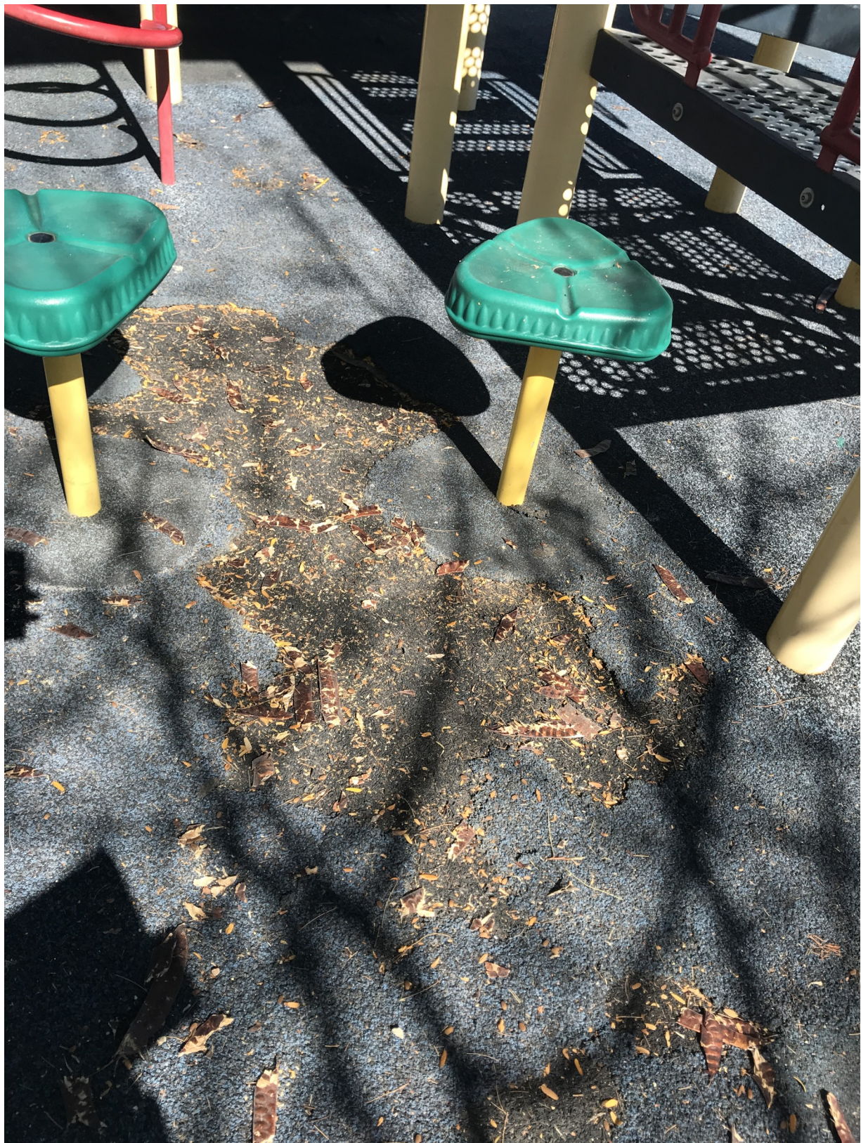
Figure 5. Worn out, Weathered, padded safety surface
