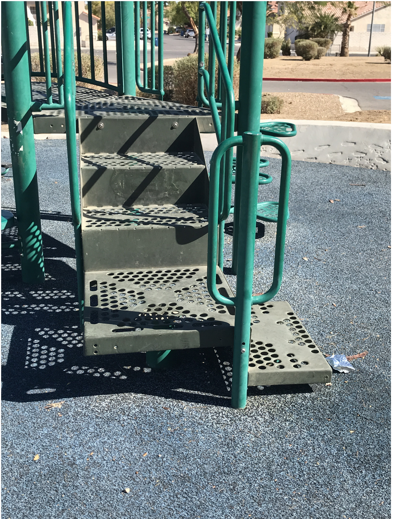
Figure 6. Age-appropriate height and guard rails to prevent falls
